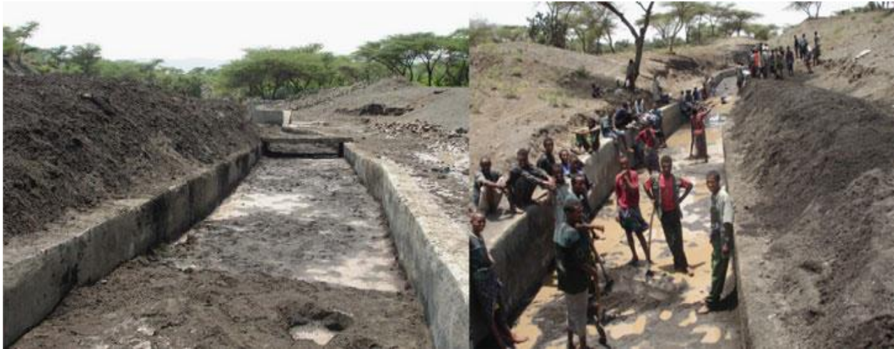
Fig. 7. Sedimentation problem in Fokisa, Tigray, Ethiopia (Gebreegziabher Embaye et al., 2008).
